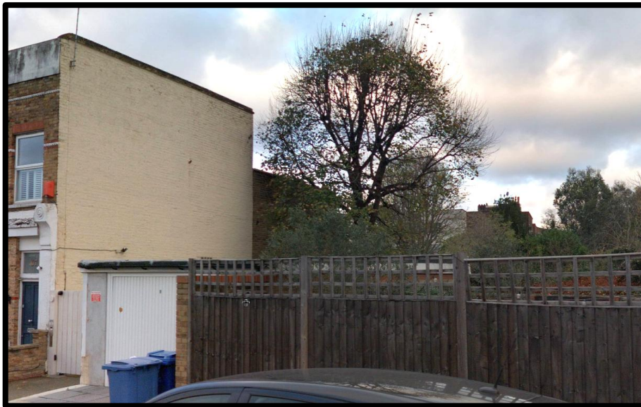
Side return wall of 67 Upland Road
